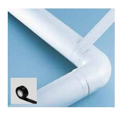
Wind the tape tightly around the joints on the straight sections...
