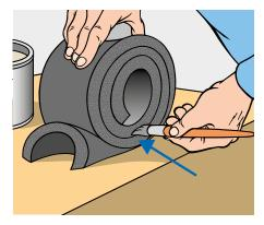
When attaching the two surfaces, press them together firmly with your fingers, starting at the far ends, then the centre and lastly along the intermediate points to avoid an irregular joint.
