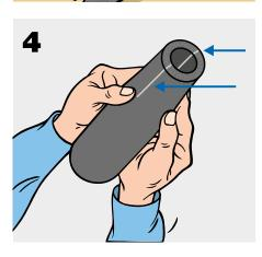
After positioning it on the pipe, glue the edges of the lengthwise cut with K-FLEX® glue and bond the edges of the sleeving to the other two sections of tubing.
