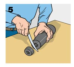
Take a piece of K-FLEX® the same diameter as the larger of the two pipes, and cut it slightly longer than the space left between the two sections of tubing already in place.
