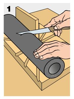
After letting the glue dry, cut the rightangled section along its length on the inside.
