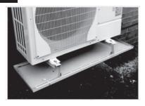
Place the outdoor unit onto the bracket leaving enough room for air circulation and fix.
